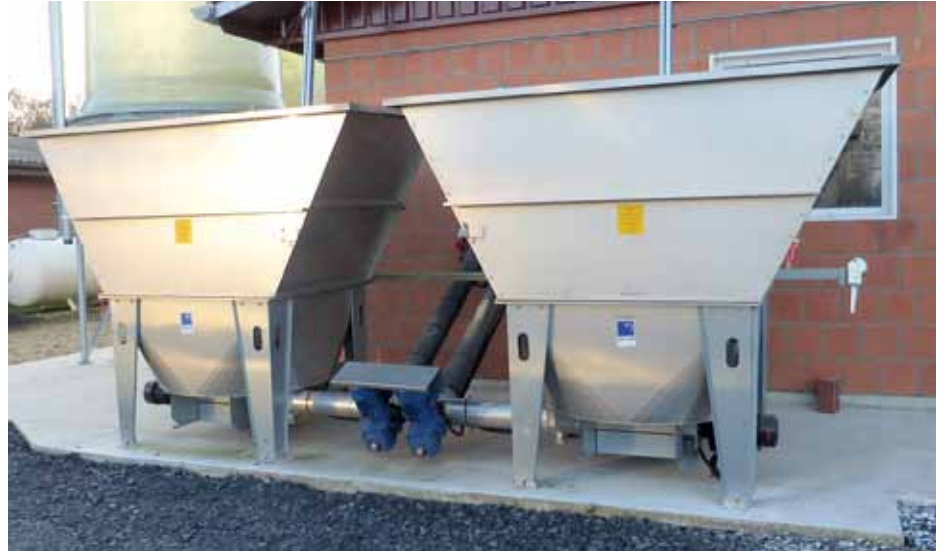
2 UNI-Dos model 45s made from stainless steel with 3.2 m 3 storage volume, horizontal discharge screw model 160, stainless steel cover with hand crank
